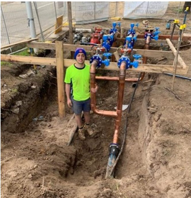
Year 11 Plumbing student Laurence Nardella on the Whittlesea nursing home job.
